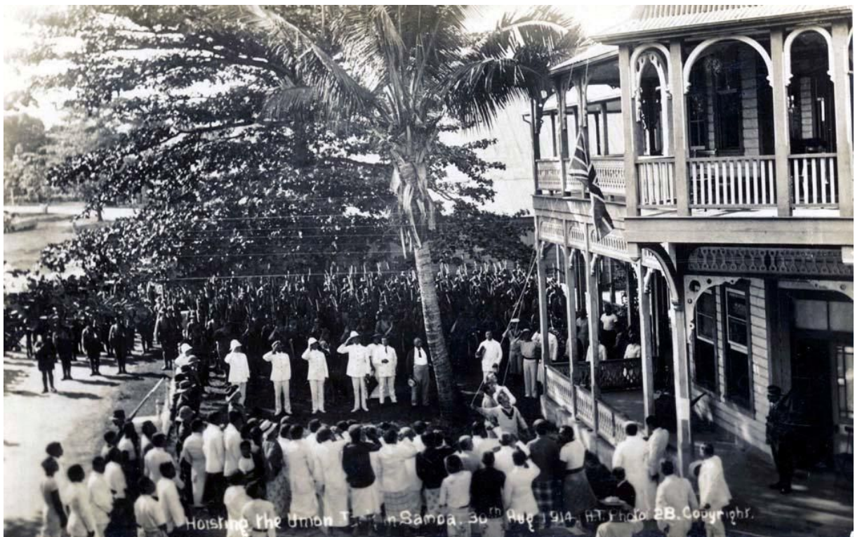
Hoisting the Union Jack in Samoa 1914.
